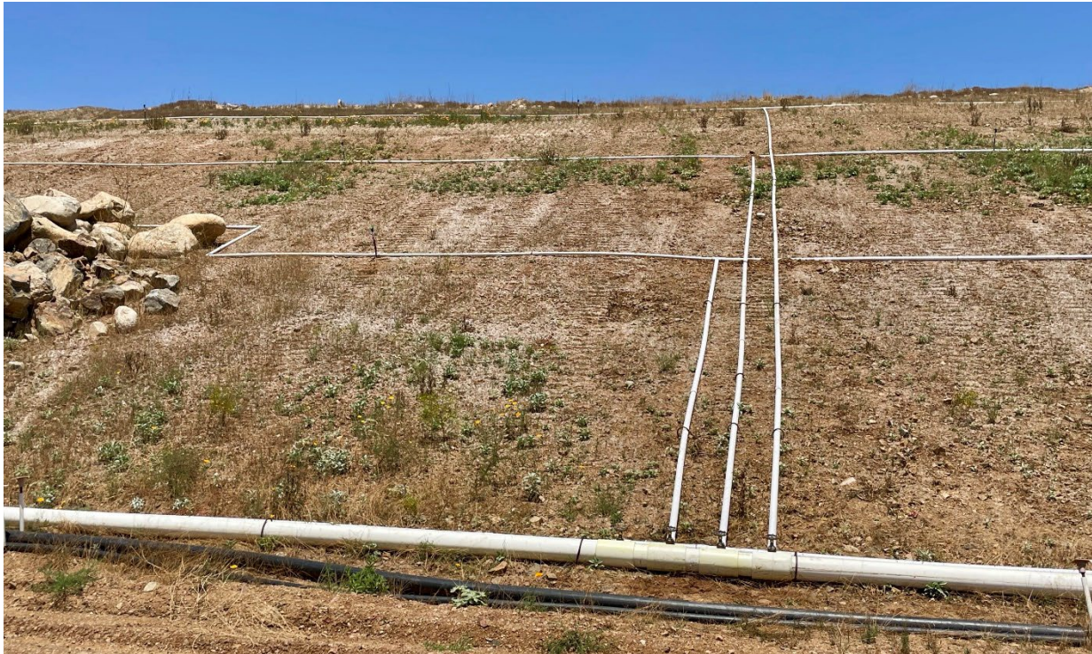
Photograph 18. A rock outcrop and irrigation system on Phase D1, June 22, 2023.
