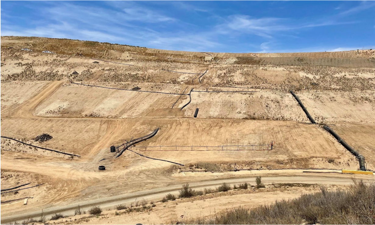
Photograph 9. Phase C1 with recent repair work, July 2022.
