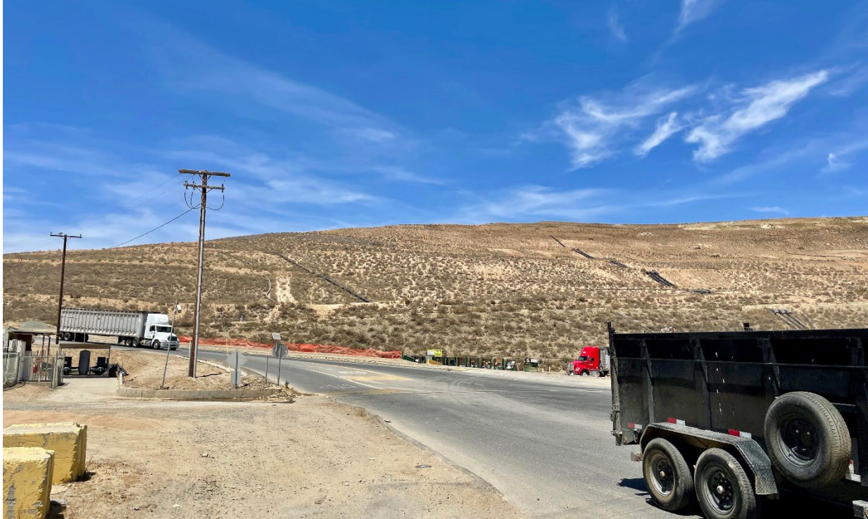
Photograph 5. The west end of the landfill, July 20, 2022.
