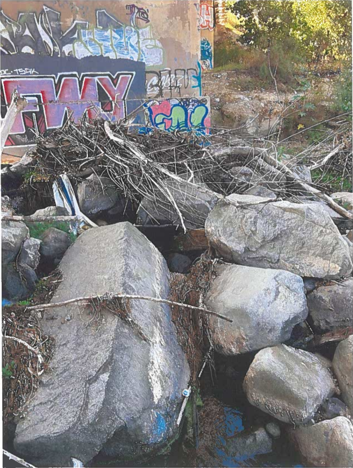
Picture 8: Channel Invert
