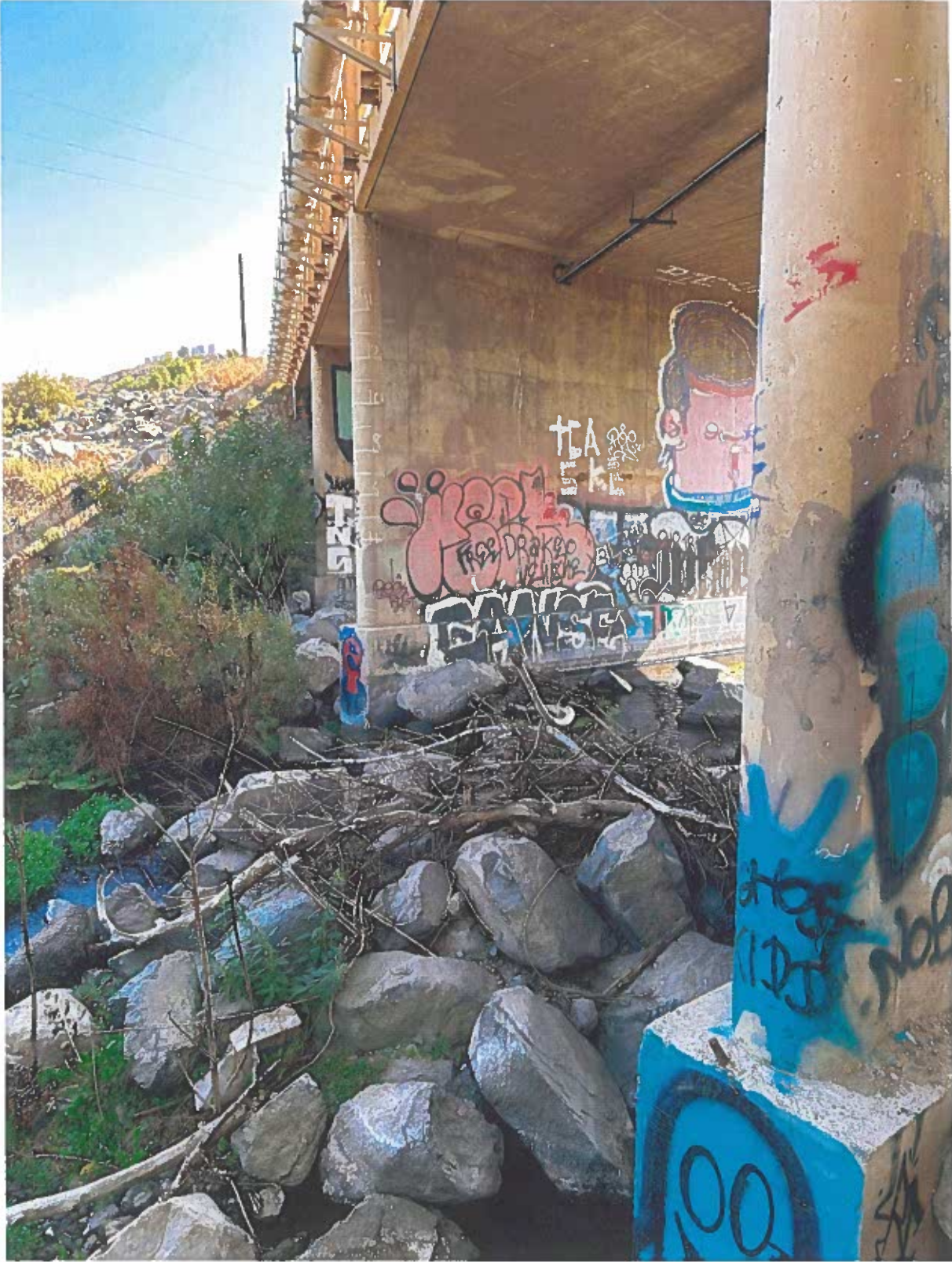
Picture 7: Channel Invert
