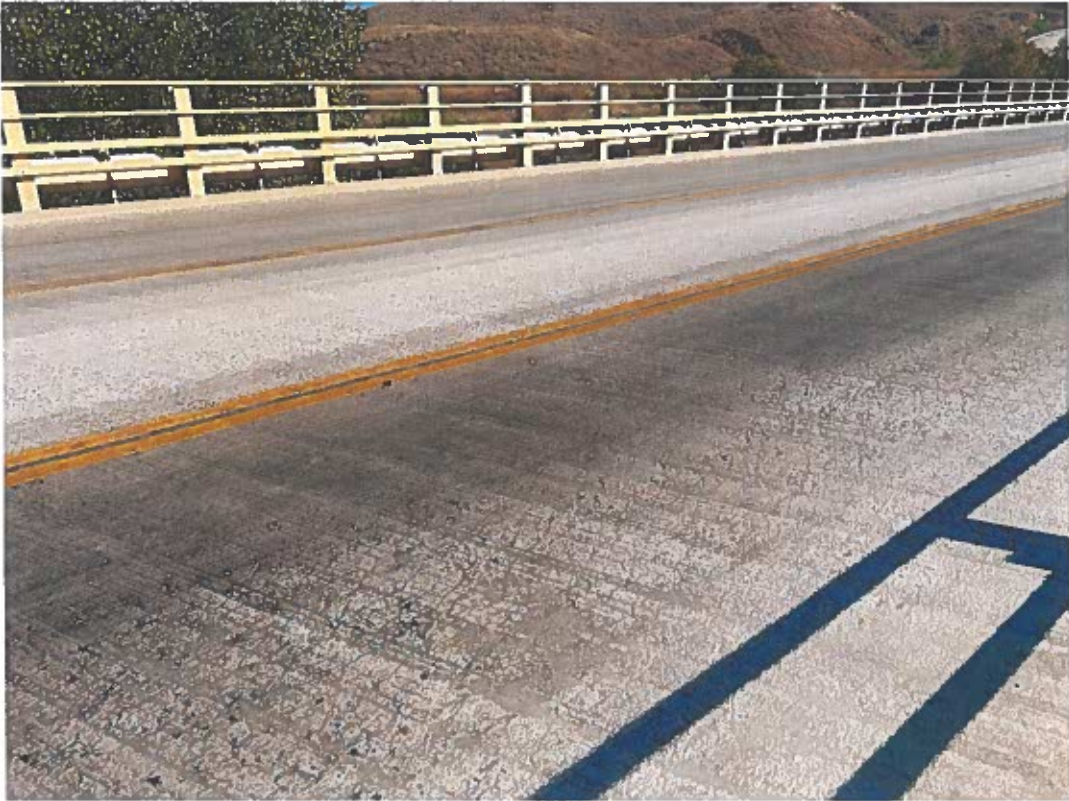
Picture 1: Concrete Bridge Deck with Methacrylate Deck Treatment
