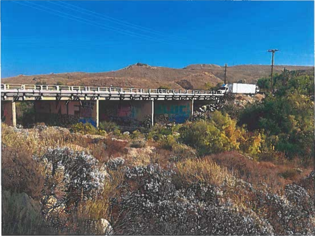
Picture 4: South Bridge Elevation
