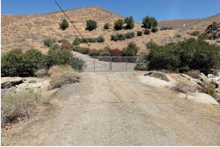
Photo 1 Pond 4 gate and fencing
