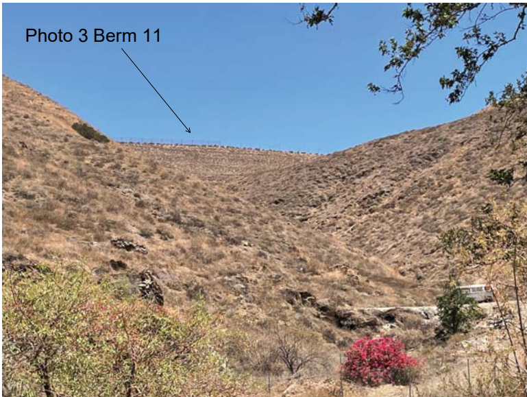
Photo 4 View of landfill from west of 1-15
