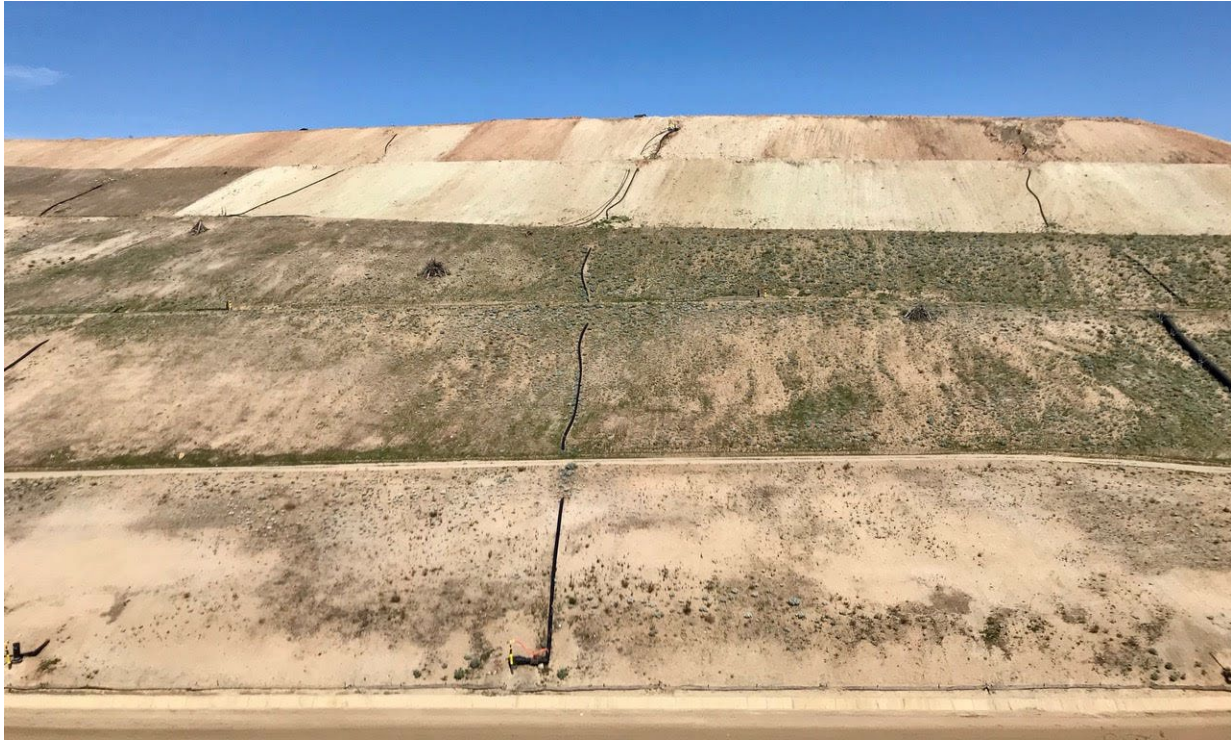
Photograph 5. Moving west, Phase C1, March 2021.
