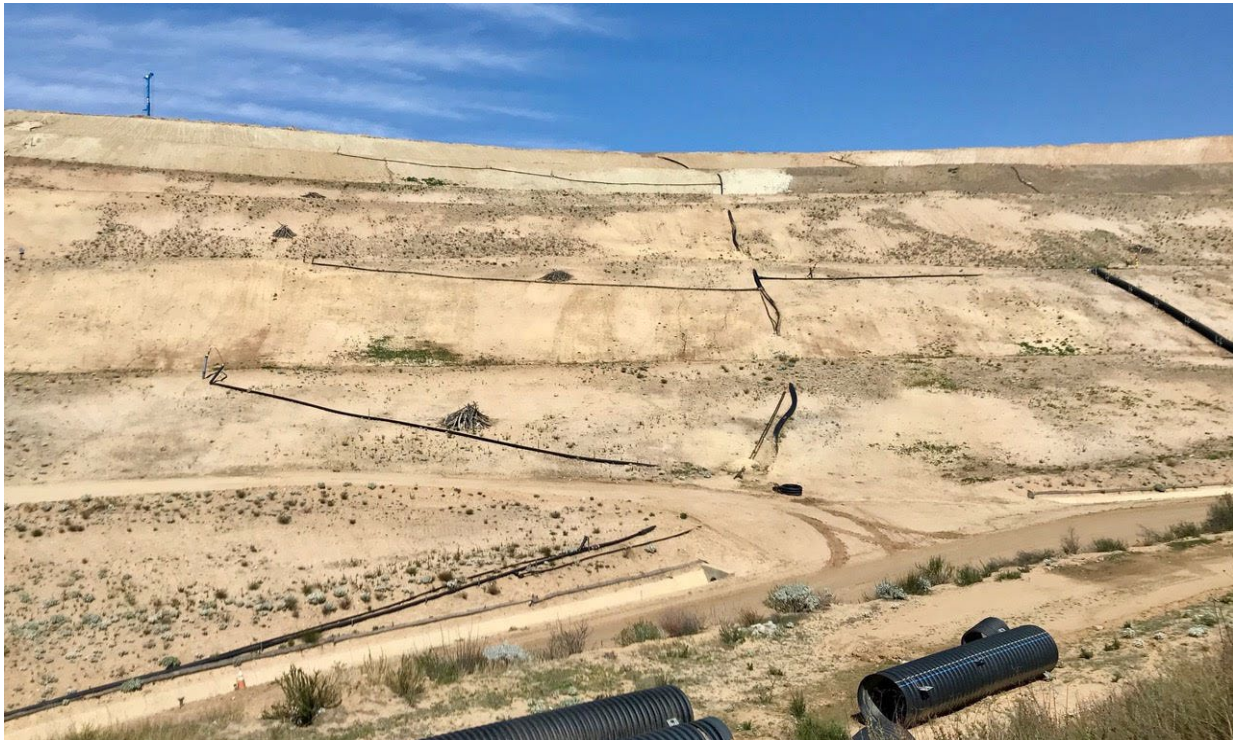
Photograph 9. Four slopes of Phase C1, March 2021.
