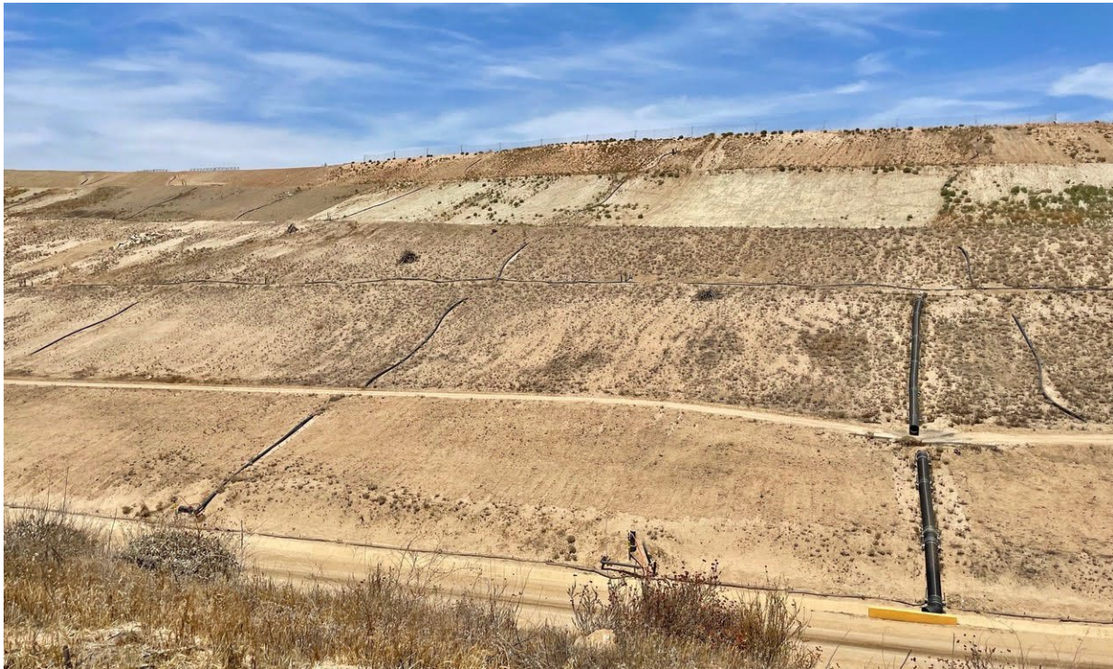
Photograph 6. Moving west, Phase C1, July 2022.
