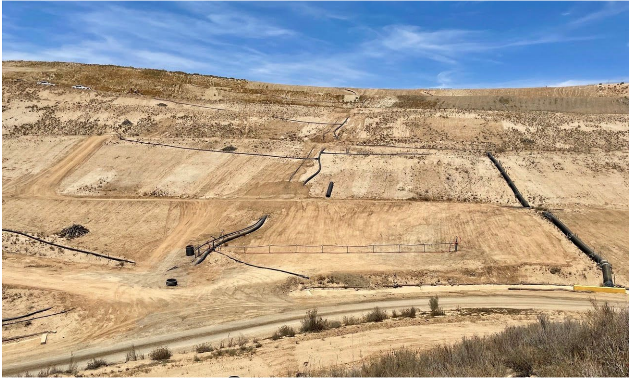
Photograph 10. Four slopes of C1 with trucks above the top slope, July 2022.
