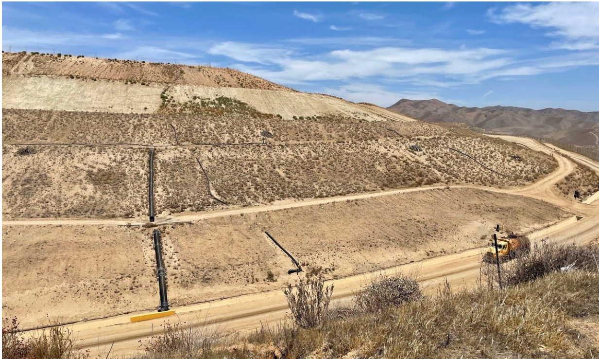
Photograph 4. The eastern part of Phase C1, July 2022.
