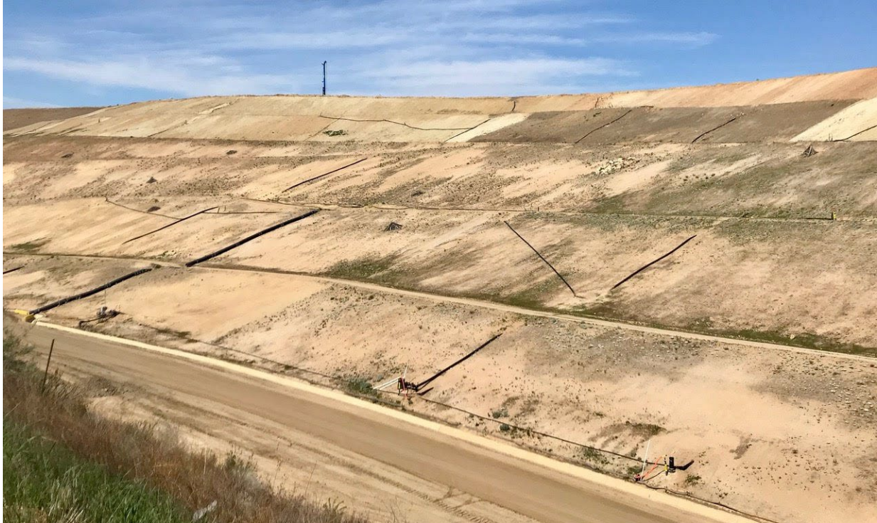
Photograph 7. The center of Phase B1, March 2020.
